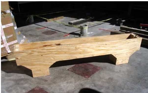
Figure 12. Wooden mold Pier Cap Beam.
